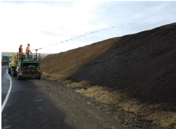
Figure 8. Hydraulically Applied Biotic Soil Amendment
