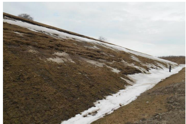
Figure 3. Well-vegetated slope sloughing within six months
