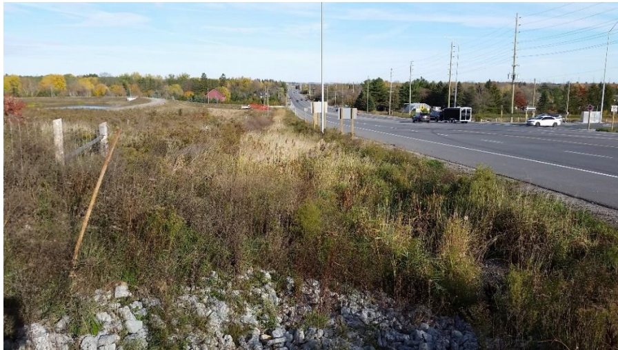
Figure 17: Stable, high performance conveyance structure utilizing TRM technology
