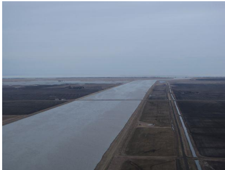
Figure 3: Spring, 2011 Failsafe on west levee (left) at the bend in the structure
