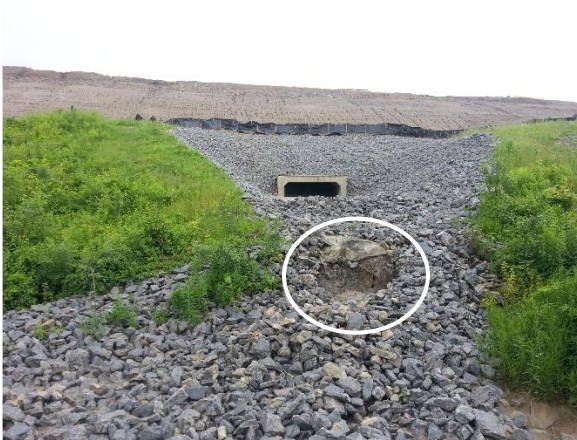
Figure 15: Storm flow out of a 1.5m high box culvert conveyed the riprap armour and ripped the geotextile.
