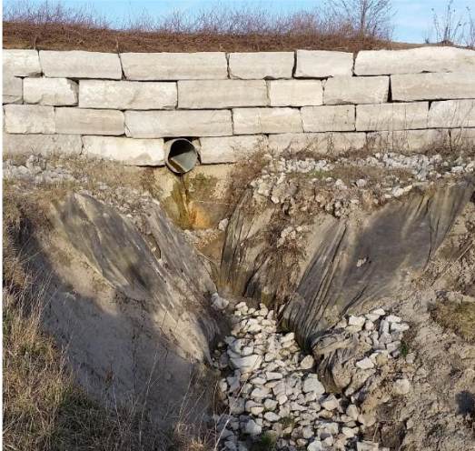
Figure 12: Apparent storm flow ‘catastrophic failure’
