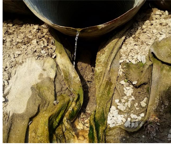
Figure 14: Persistent nuisance flow cause of failure
