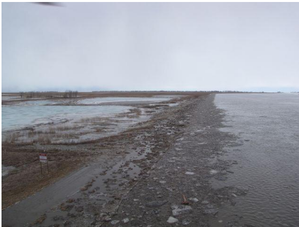
Figure 7: Spring, 2011 Failsafe overtopping
