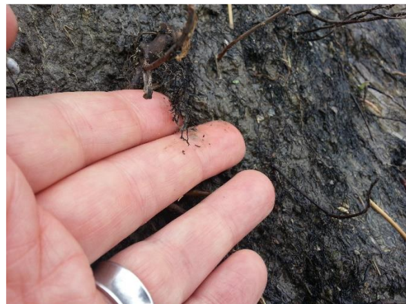
Figure 16: Grade remained stable because of remnant shrub rootzone left in place below the geotextile.
