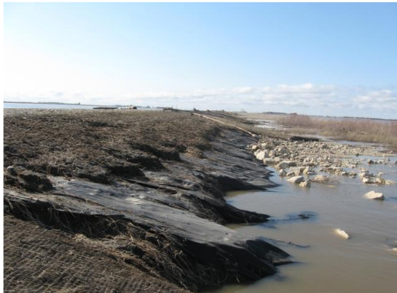
Figure 11: Spring, 2009 300mm (1ft) riprap conveyed in overtopping, adjacent TRM in the foreground performed
