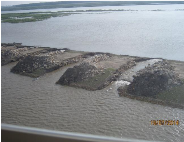
Figure 9: July, 2014 Mechanical breaching of TRM on failsafe slope
