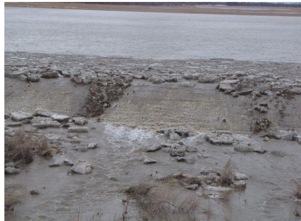
Figure 8: Spring, 2011 Ice overtopping detail
