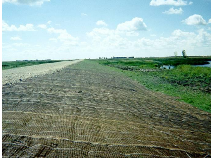
Figure 4: Summer, 1997 Failsafe armoured utilizing TRM technology
