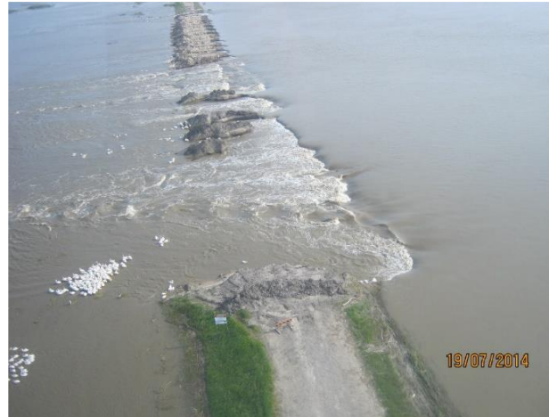
Figure 10: July, 2014 Failsafe left, wet side right
