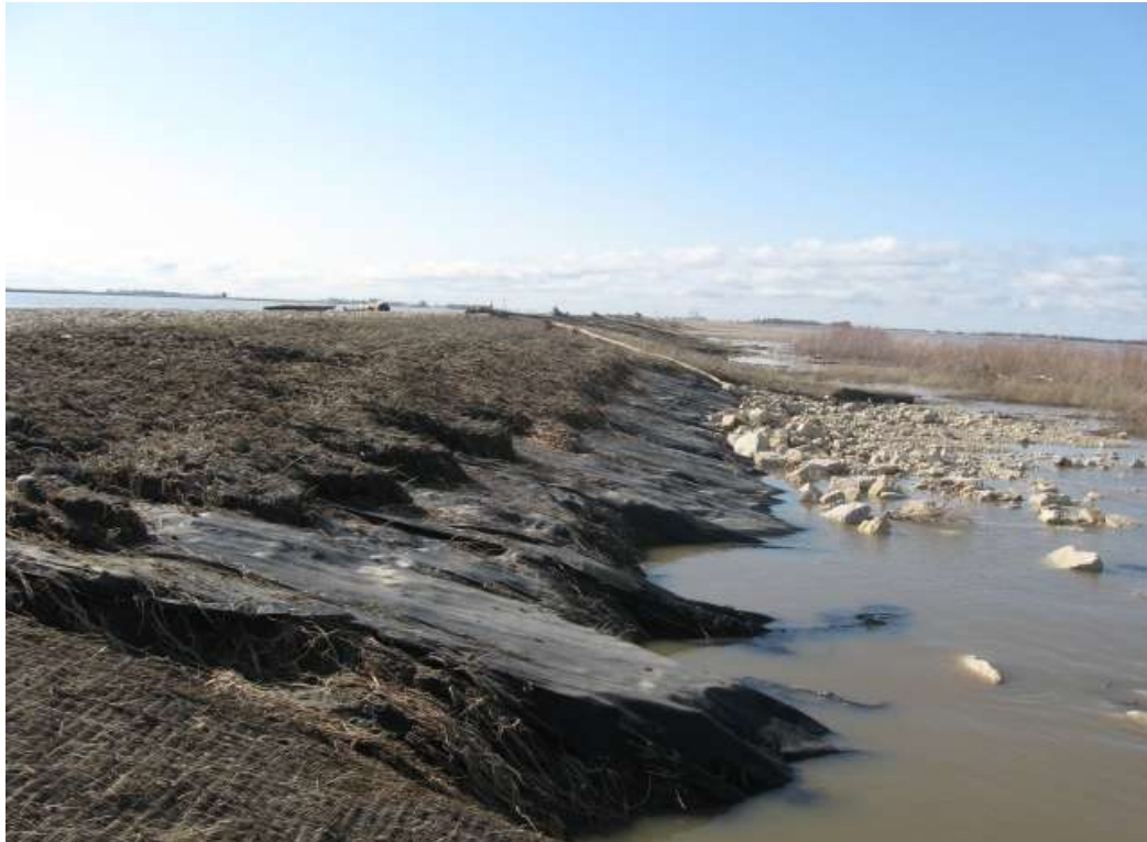
Spring, 2009 300mm rock armour conveyed in overtopping, adjacent TRM in the foreground performed
